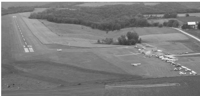
The Rushford Airport Viewed from the Air
