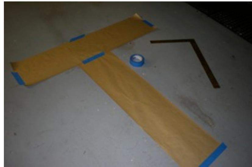
Make sure to tape the paper so it will not shift during the measurement process.
