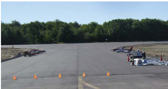
Brand New Pavement at Maine!
